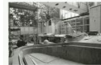
The Vera List Courtyard of The New School Under Construction (NS040101_000488)
