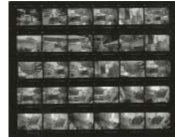
The Vera List Courtyard of The New School Under Construction (NS040101_000519)
