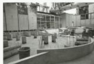
The Vera List Courtyard of The New School Under Construction (NS040101_000492)
