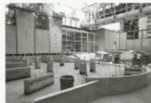
The Vera List Courtyard of The New School Under Construction (NS040101_000487)
