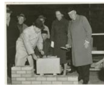
Mayor Robert F. Wagner Laying the Cornerstone for the Addition to the 66 W. 12th Street New School Building (NS040101_000402)
