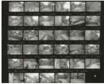
The Vera List Courtyard of The New School Under Construction (NS040101_000525)
