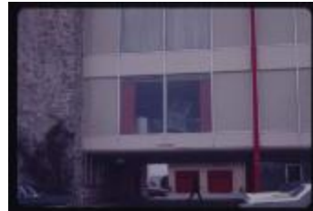
Modular Environmental Structural System, or M.E.S.S., in Second Floor Building Window as Seen from Street (KA0123_b01_f13_s23)
