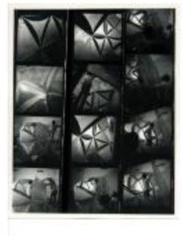
Construction of a M.E.S.S. Unit (KA0123_b01_f09_01)
