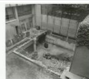
The Vera List Courtyard of The New School Under Construction (NS040101_000491)
