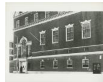
Building Façade at 150 West 85th Street (MA040101_000079)
