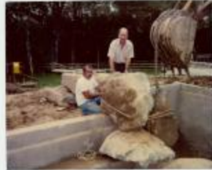
Polaroid of Ginsberg Project Rock Installation (KA0119_b18_f06_06)
