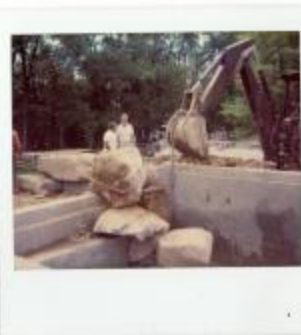
Polaroid of Ginsberg Project Rock Installation (KA0119_b18_f06_02)
