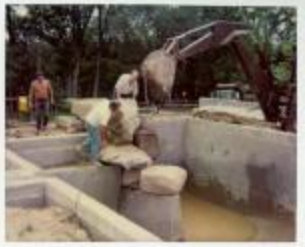
Polaroid of Ginsberg Project Rock Installation (KA0119_b18_f06_05)
