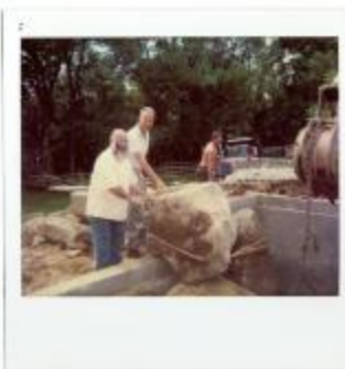
Polaroid of Ginsberg Project Rock Installation (KA0119_b18_f06_01)
