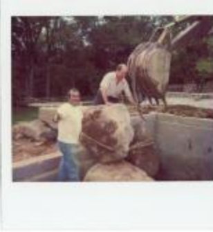
Polaroid of Ginsberg Project Rock Installation (KA0119_b18_f06_03)
