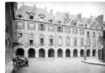
Exterior of Paris Ateliers (PIC03002_b17_f16_02)
