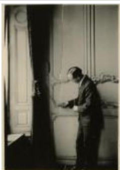
Man Inspecting Wall Paneling (PIC03002_b17_f15_11)
