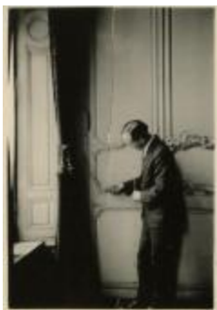
Man Inspecting Wall Paneling (PIC03002_b17_f15_11)
