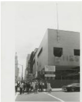
Graduate Center of the New School for Social Research Construction (NS040101_000178)
