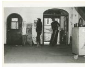
Renovations at 150 West 85th Street (MA040101_000030)
