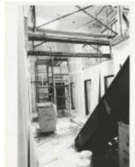
Construction at 150 West 85th Street (MA040101_000034)
