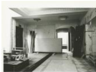
Atrium Renovations (MA040101_000033)
