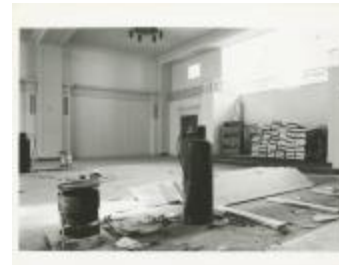
Renovations at 150 West 85th Street (MA040101_000031)
