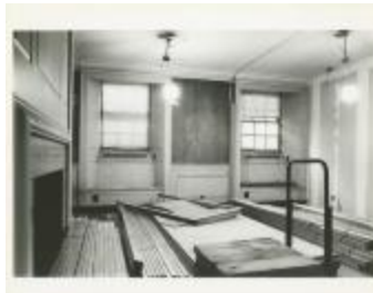
Renovations at 150 West 85th Street (MA040101_000026)
