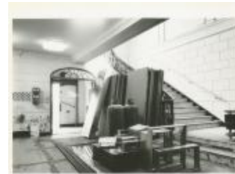
Interior Staircase Renovations at 150 West 85th Street (MA040101_000035)
