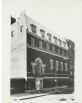
Building Facade at 150 West 85th Street (MA040101_000050)
