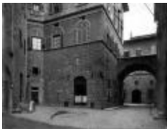
Exterior, Florence Facilities, New York School of Fine and Applied Art (PIC03002_b17_f14_05)
