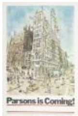
Parsons is Coming! (PIC05007-1_OSxxx1_f03_05)
