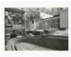
The Vera List Courtyard of The New School Under Construction (NS040101_000488)
