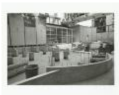
The Vera List Courtyard of The New School Under Construction (NS040101_000492)
