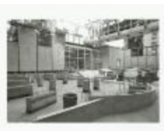
The Vera List Courtyard of The New School Under Construction (NS040101_000487)
