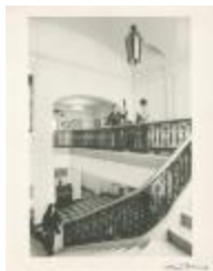
Interior Stairway at 150 West 85th Street (MA040101_000009)
