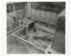
The Vera List Courtyard of The New School Under Construction (NS040101_000491)
