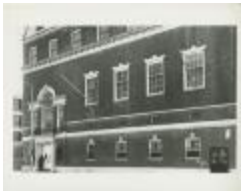
Building Façade at 150 West 85th Street (MA040101_000079)
