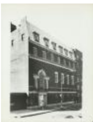
Building Facade at 150 West 85th Street (MA040101_000050)
