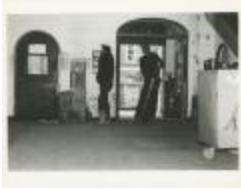
Renovations at 150 West 85th Street (MA040101_000030)
