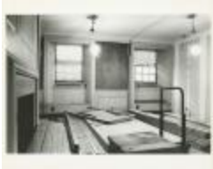
Renovations at 150 West 85th Street (MA040101_000026)
