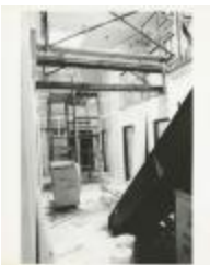
Construction at 150 West 85th Street (MA040101_000034)
