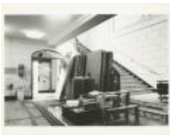
Interior Staircase Renovations at 150 West 85th Street (MA040101_000035)
