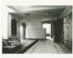
Atrium Renovations (MA040101_000033)
