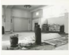
Renovations at 150 West 85th Street (MA040101_000031)
