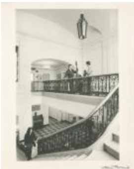
Interior Stairway at 150 West 85th Street (MA040101_000009)
