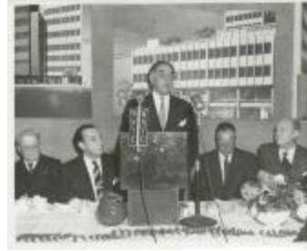
Albert Mayer Speaking at Cornerstone Laying Luncheon for Addition to 66 West 12th Street Building of The New School (NS040101_000396)
