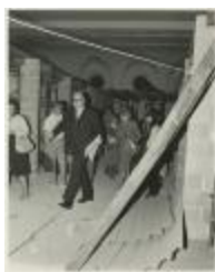
Group Touring Building Construction Site (MA040101_000087)
