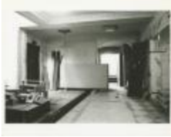
Atrium Renovations (MA040101_000033)
