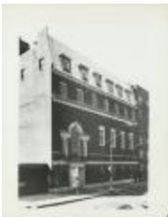
Building Facade at 150 West 85th Street (MA040101_000050)
