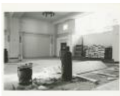
Renovations at 150 West 85th Street (MA040101_000031)
