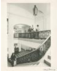
Interior Stairway at 150 West 85th Street (MA040101_000009)
