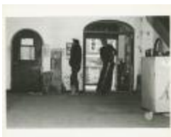
Renovations at 150 West 85th Street (MA040101_000030)
