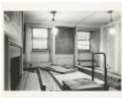
Renovations at 150 West 85th Street (MA040101_000026)
