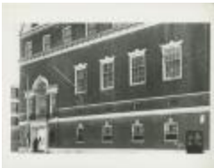
Building Facade at 150 West 85th Street (MA040101_000079)
