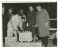
Mayor Robert F. Wagner Laying the Cornerstone for the Addition to the 66 W. 12th Street New School Building (NS040101_000402)
