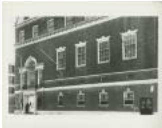
Building Façade at 150 West 85th Street (MA040101_000079)
