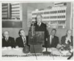
Stanley M. Isaacs Speaking at Cornerstone Laying Luncheon for Addition to 66 West 12th Street Building of The New School (NS040101_000394)
